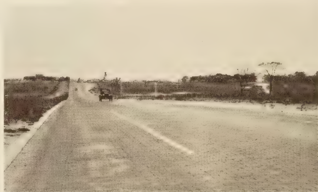
40-FOOT BRICK PAVEMENT NORTH OF AKRON, OHIO
